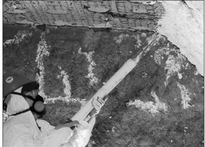
Foamfrax Installation
